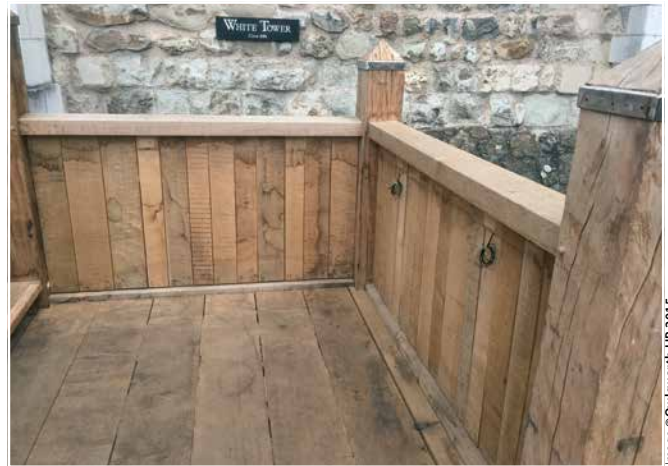
The lower landing showing the quarter sawn oak boards of the balustrade.
